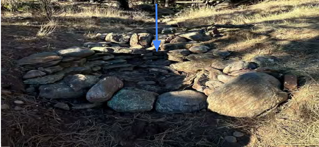
Zuni Bowl constructed by HPWA seasonal crews in Sapello (Fall 2023).
