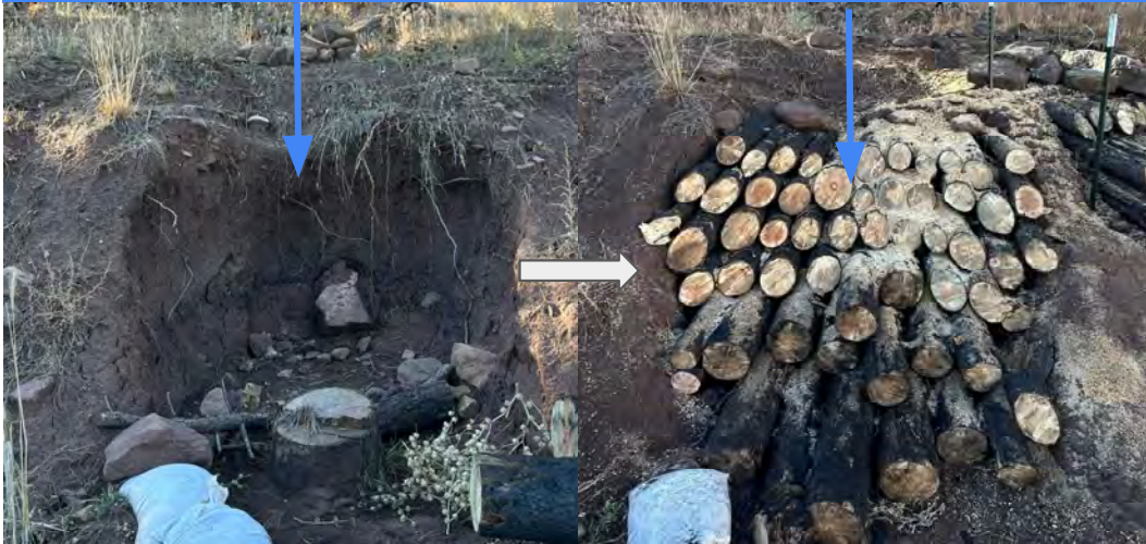
Head-cut (left) formation addressed by Log Step Down (right) constructed by HPWA Seasonal Crews in Sapello (Fall 2023).
