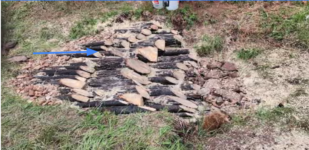
Log Step Down constructed by seasonal crews during training in Gallinas (Summer 2023).
