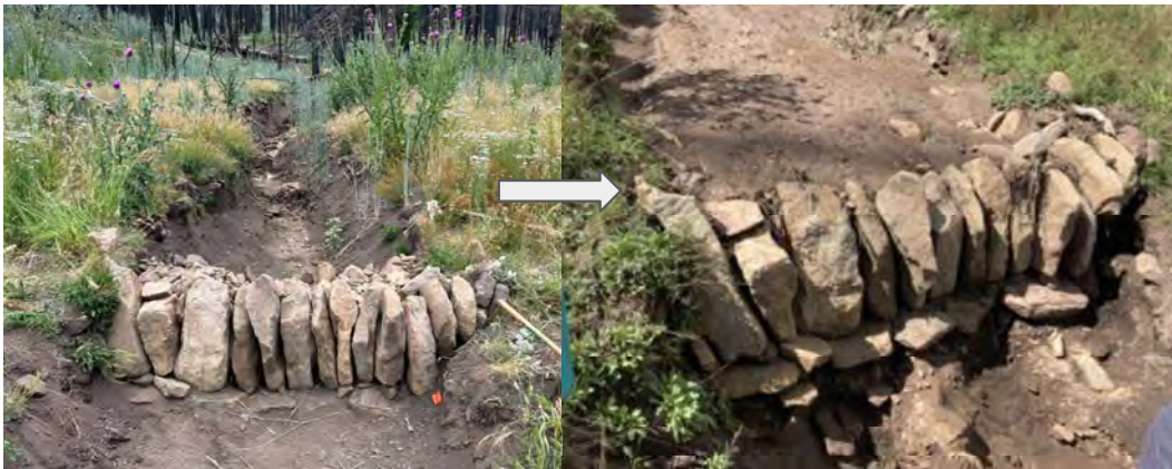
One Rock Dam constructed by HPWA seasonal crews in Sapello before (left) and after (right) filling up with sediment (Summer 2023).
