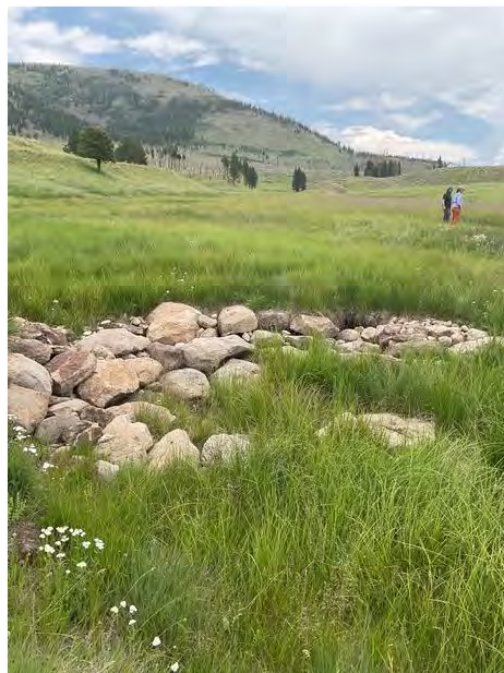
Figure 3-6. Undercutting or piping through the rocks is seen on the far side of the Zuni Bowl wall on the right. Santa Rosa #6, Object ID 55 in survey. Location: -106.5974051, 35.92597653. Looking toward valley left.
