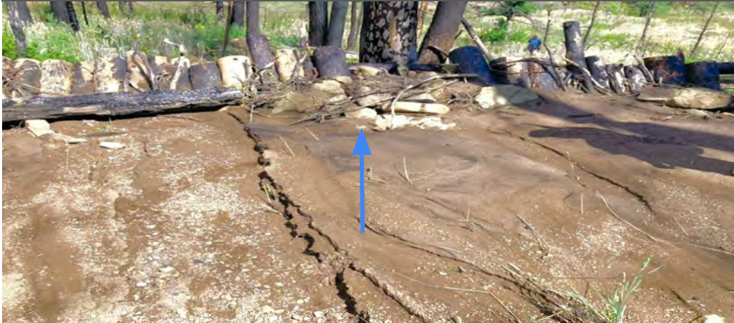
Trash Rack filled with sediment constructed by HPWA and FSG seasonal crews in Sapello (Summer 2023).
