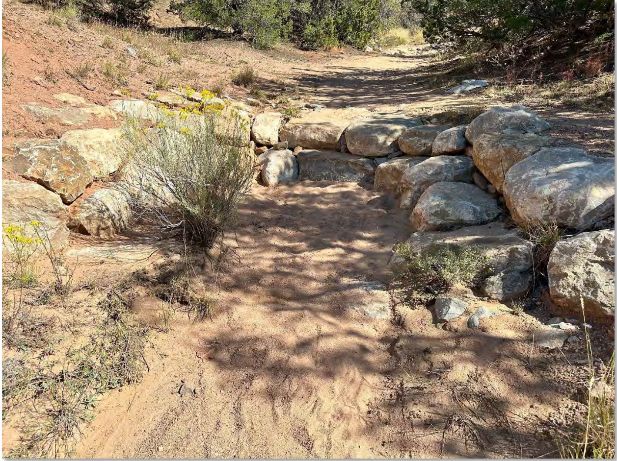
Figure 4-5. Zuni Bowl in the arroyo at Santa Fe Botanical Gardens. Photo taken on a clear day prior to the field trip. Location: -105.928595, 35.665349.
