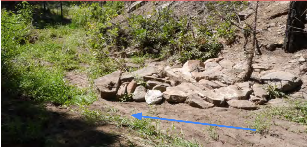
Baffle constructed by HPWA seasonal crews in Sapello (Summer 2023).
