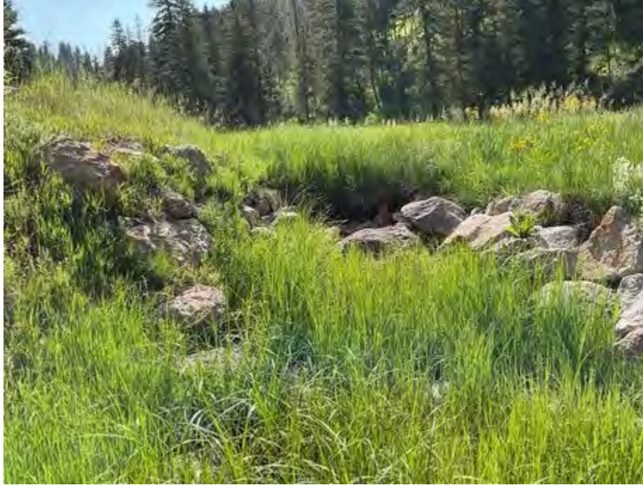
Figure 3-4. Example of some rocks dislodged or broken. Rocks were displaced from the Zuni Bowl Pour-Over shown in the center of the photo. Sulphur Creek #2. Object ID 51 in survey. Location: -106.6014258, 35.9241155. Photo looking upslope.
