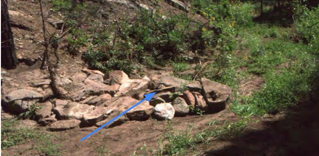
Baffle constructed by HPWA seasonal crews in Gallinas (Summer 2023).
